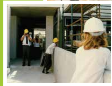
KELLY STREET Construction begins
