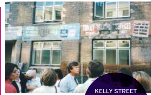
KELLY STREET The fire-ravaged Dalgety's woolstore in Kelly Street
